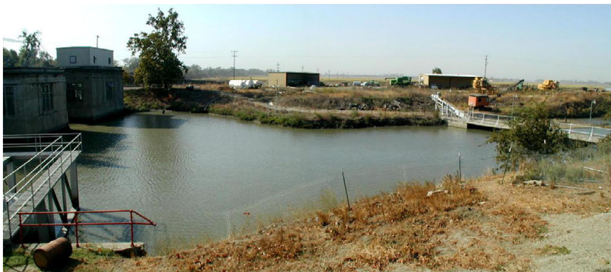
Karnak Pumping Plant Forebay
