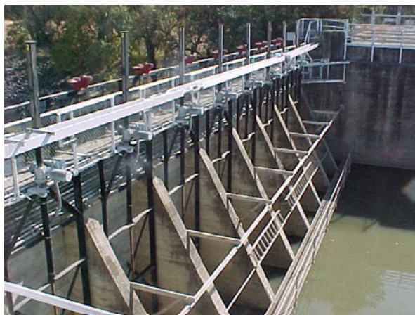
Colusa Basin Drain Outfall Structure
