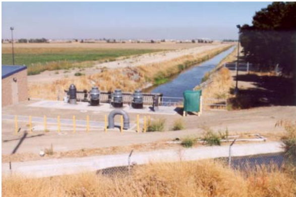
RD 1000 Pumping Plant 3
