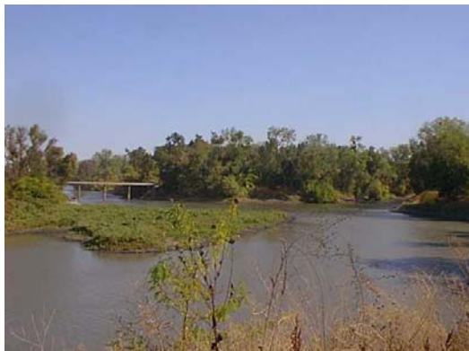
Sutter Bypass at Karnak Pumping Plant Discharge and Beginning of the Sacramento Slough
