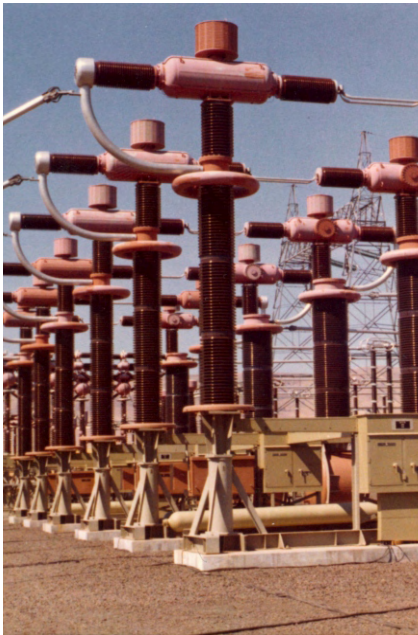
Hydroelectric power generation
