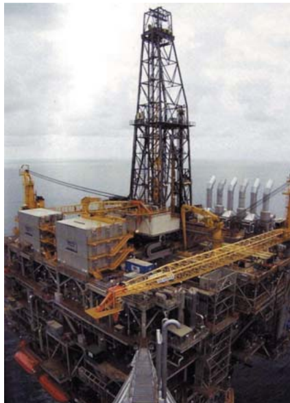
The Holstein oil and gas development is located approximately 150 miles south of New Orleans. The field is being developed using a Production Drilling and Quarters (PDQ) truss spar, permanently moored in 4,350 feet of water. Photo courtesy of BP Exploration & Production.
