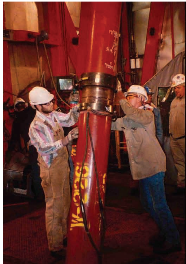
J-lay pipeline welding and weld inspection operations.
