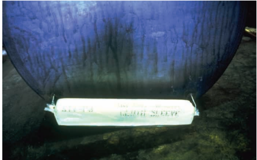
Sacrificial anode on a steel underground storage tank. Photo courtesy of www.epa.gov .
