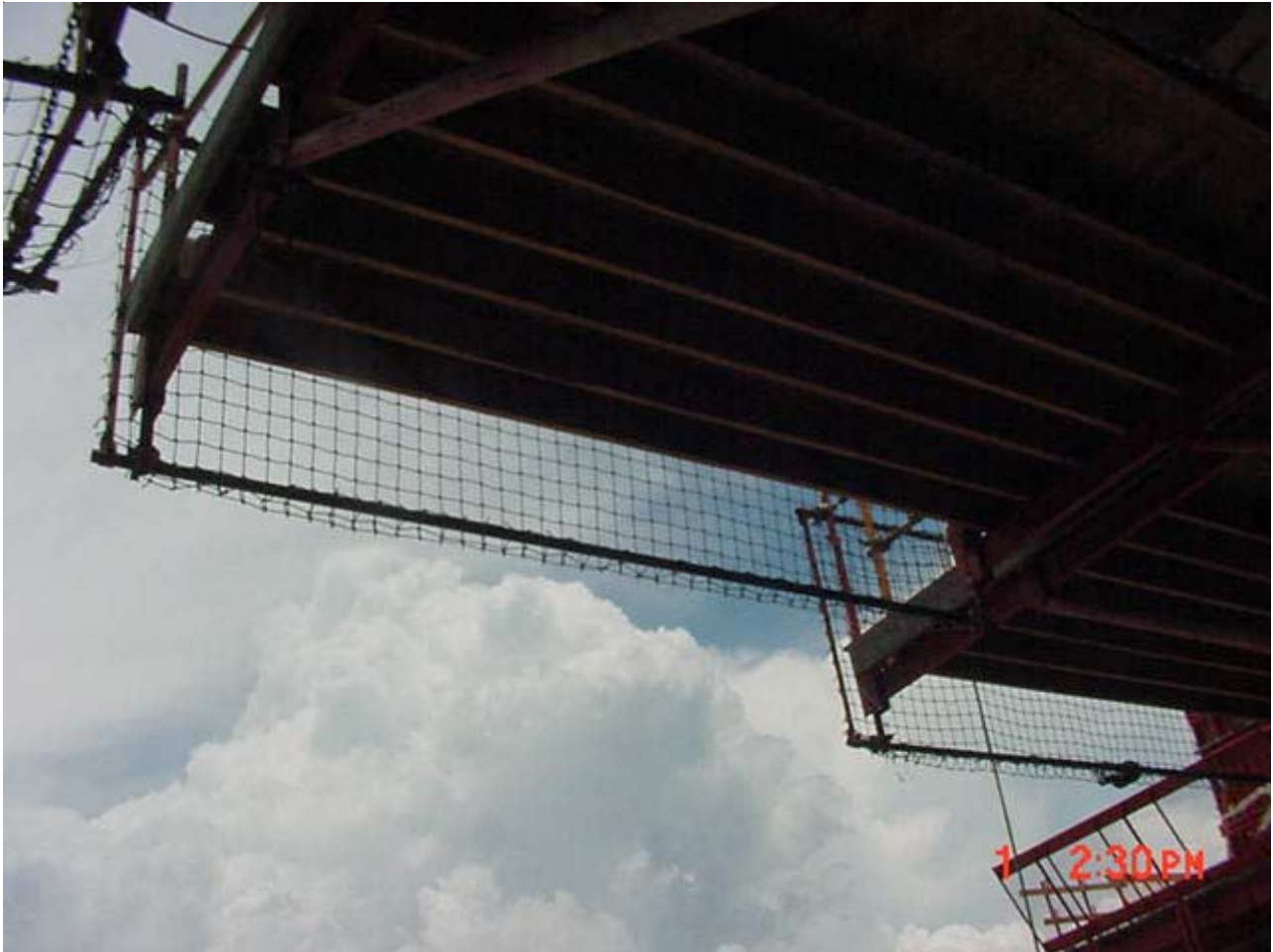
Underside of Stripping Platform showing mesh guarding.
