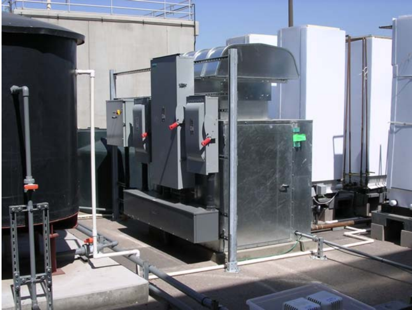
Figure 8. First tower set with steam generator and tanks.
