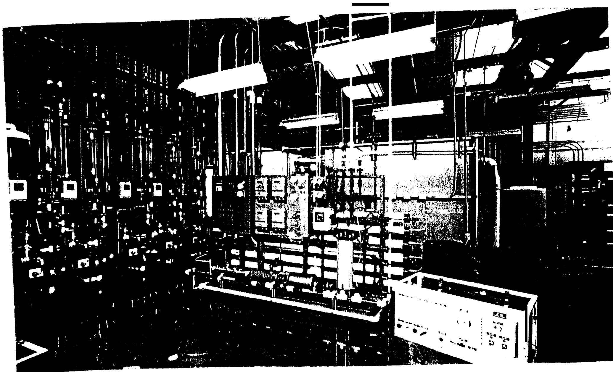
Figure 5. Photograph: Process Treatment Trains.-IRWD
