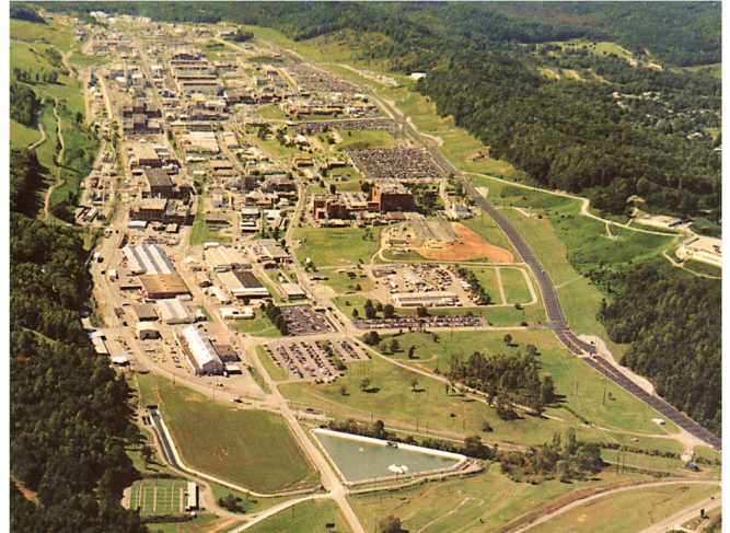
The 825-acre Y-12 plant is located 2 miles south of downtown Oak Ridge and is separated from the main residential areas of Oak Ridge by Pine Ridge.
