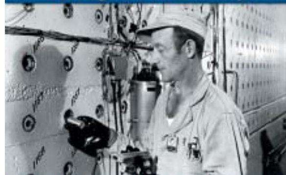
L.P. Jernigan inserts slugs of reactor fuel into a fuel channel.
