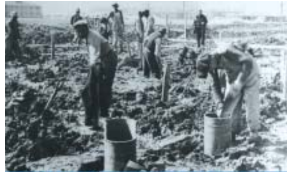
Workers toil together to help build the Oak Ridge National Laboratory.
