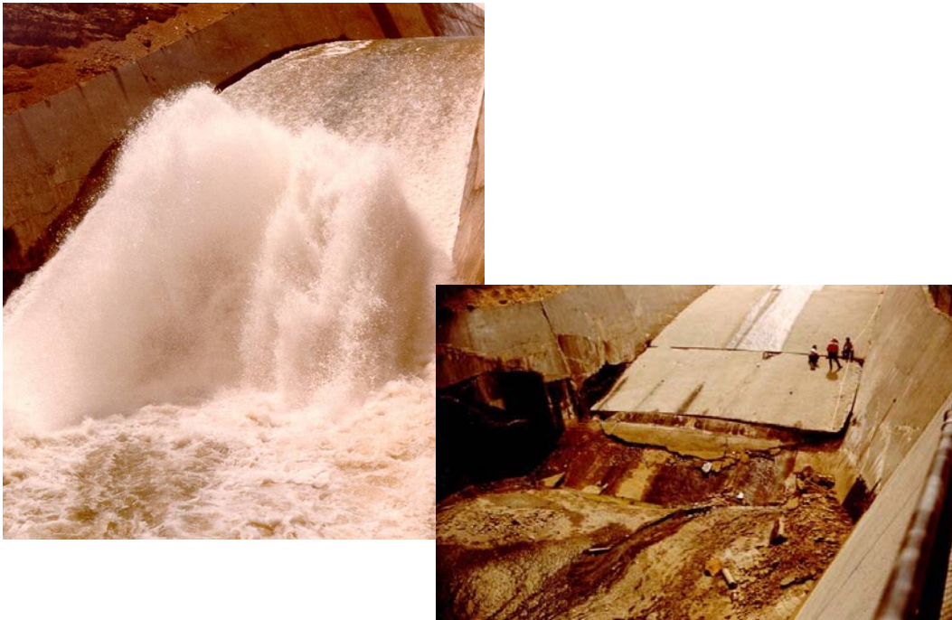
Figure 2. —If flow is allowed to continue, slabs may lift resulting in wild spray and rooster tails, and when the water recedes - slabs are damaged or missing.
