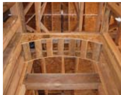
Figure III-14. Framing box-downs are not air-sealed
