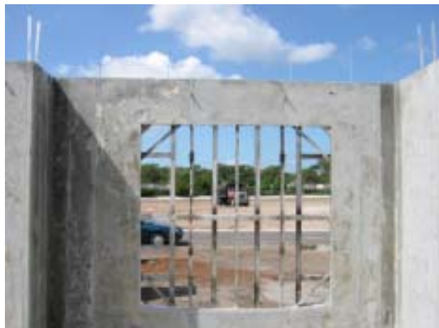
Figure II-18. Wall forms stripped, with window form in place
