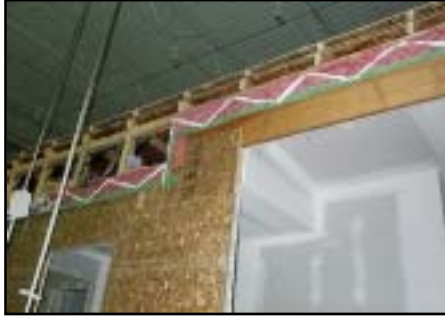
Figure I-43. Batt insulation for sealing marriage wall
