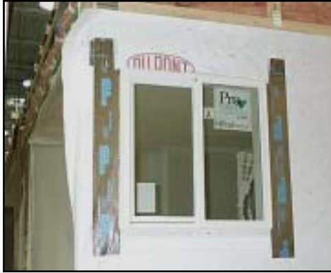
Figure I-47. Manufacturer's recommended window flashing detail
