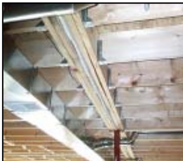
Figure I-45. Expandable spray foam at marriage wall
