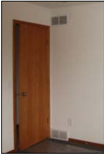
Figure I-24. High and low returns in exterior walls
