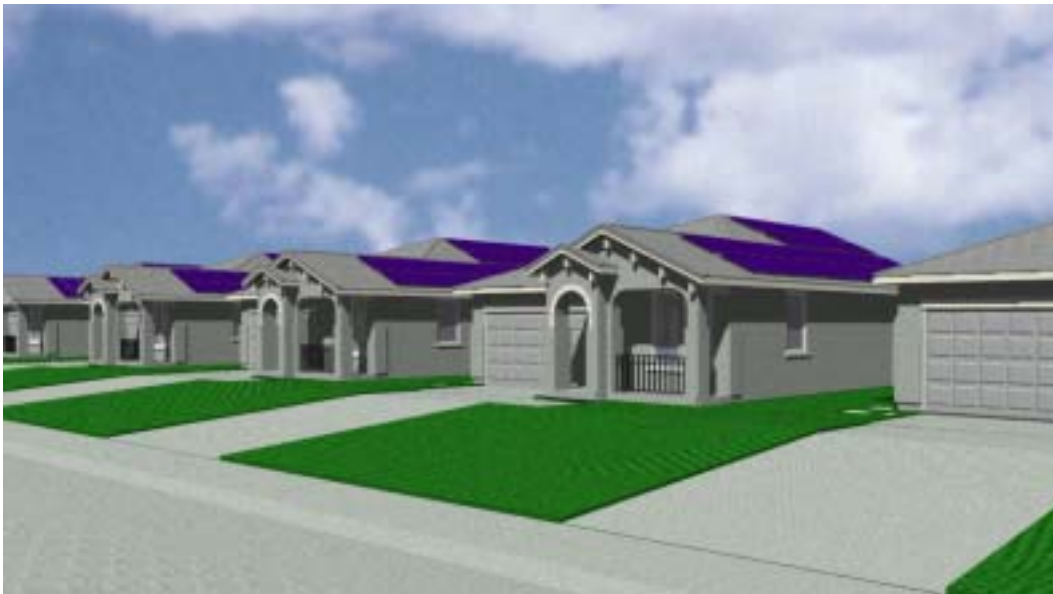
Figure III-17. Illustration of five Beazer 1330 models being offered at Roseview with 3.3-kW Sunslate PV systems
