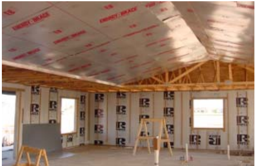
Figure III-10. CARB's plenum truss
