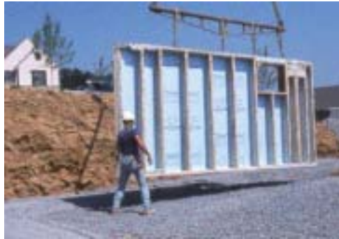
Figure I-15. Precast foundation system
