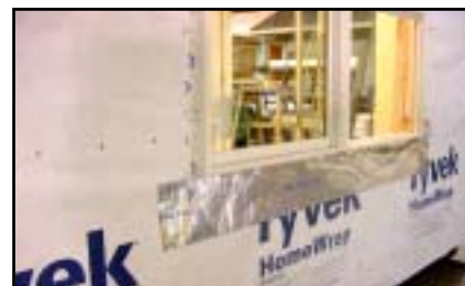
Figure I-46. Self-sealing tape at base of window
