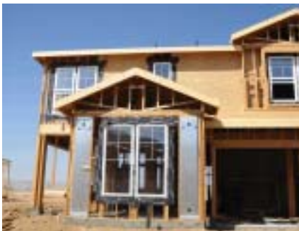
Figure III-14. Framing box-downs are not air-sealed
