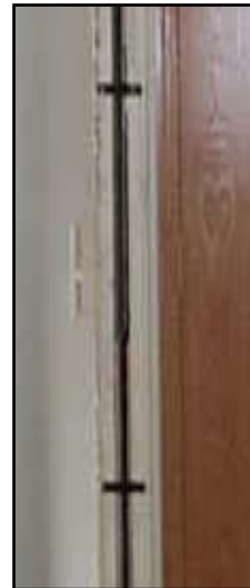
Figure I-44. Gasket seal at marriage wall
