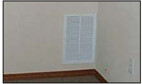
Figure I-36. First-floor low central return
