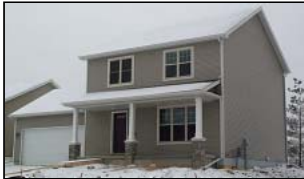
Figure I-21. Newly completed Don Simon Prototype Home
