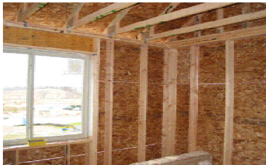
Fig. I-18. In-line framing
