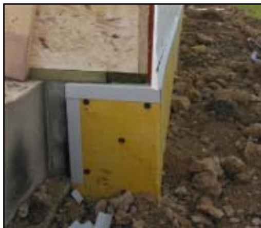
Figure I-30. Prototype foundation insulation detail
