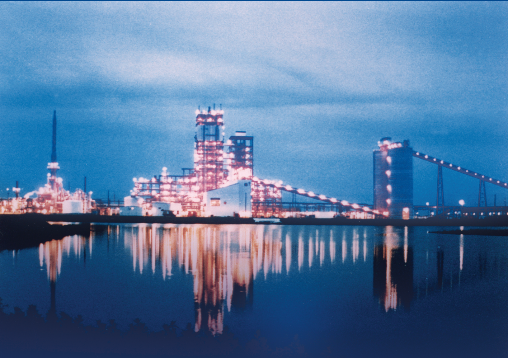
Tampa Electric Power Company's Polk Power Station at night.
