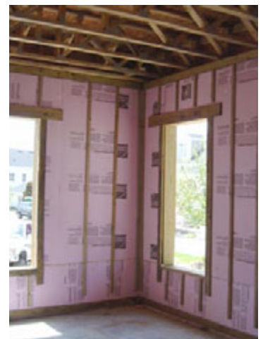
FIGURE 11: Masonry Walls with Interior Rigid Insulation
