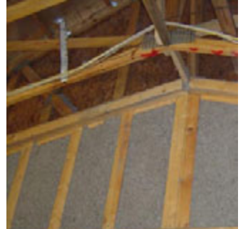
Blown-in wall insulation
