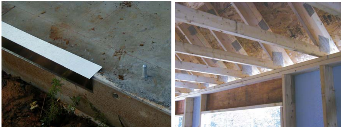
Figure 3-13. Flashing (left) and slider trusses (right)
