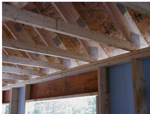
Figure 1-7. A "slider" truss
