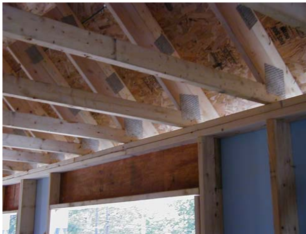
Figure 2-16. A "slider" truss
