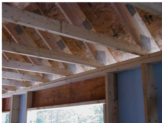
Figure 1-13. Energy trusses, also known as a “slider truss”
