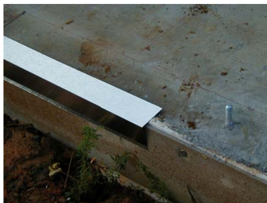
Figure 4-5. Flashing with FiberCement board
