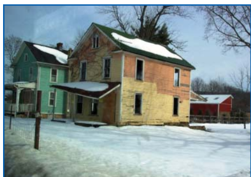
The site of the "gut rehab"
