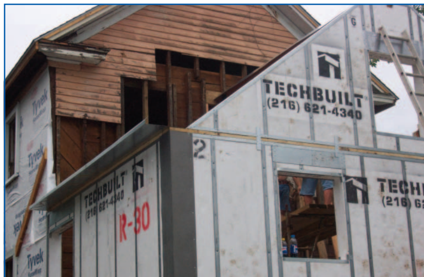
Addition construction using foam panels
