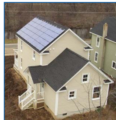
Aerial view of PV system
