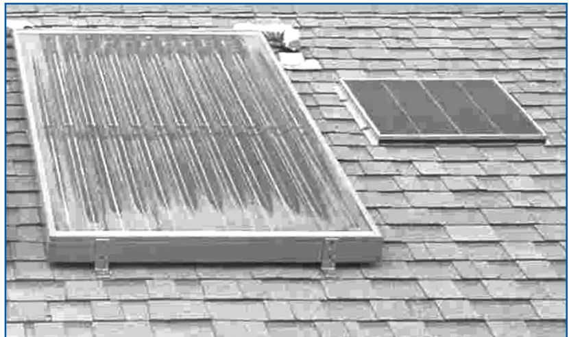
Solar thermal collector with PV panel for pump
