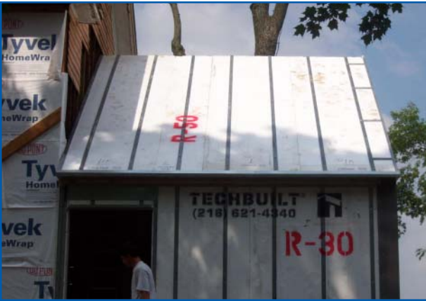
R-50 roof and R-30 wall panels
