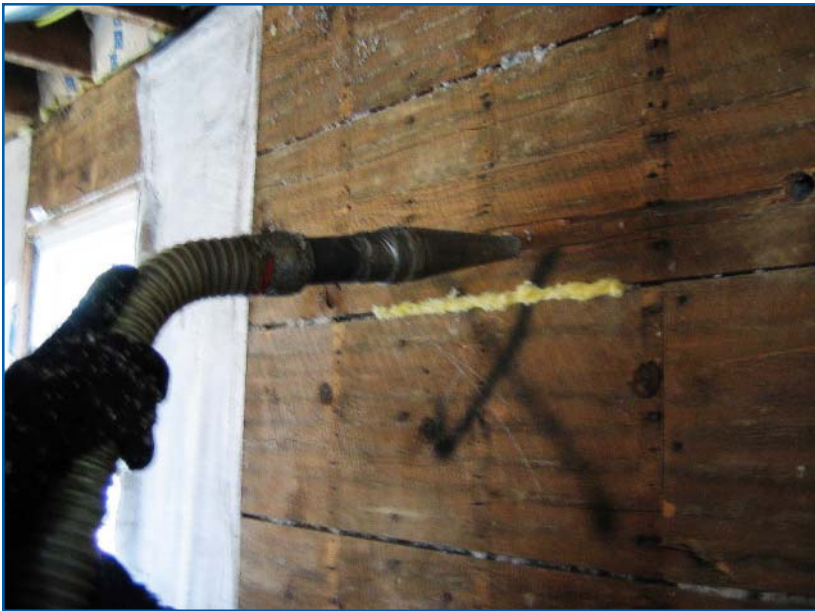
Insulation blown into wall cavities
