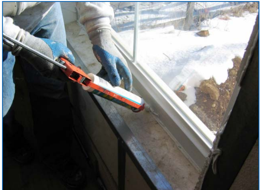
Air sealing around windows
