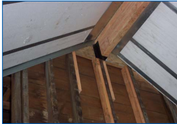
Ridge beam for roof support
