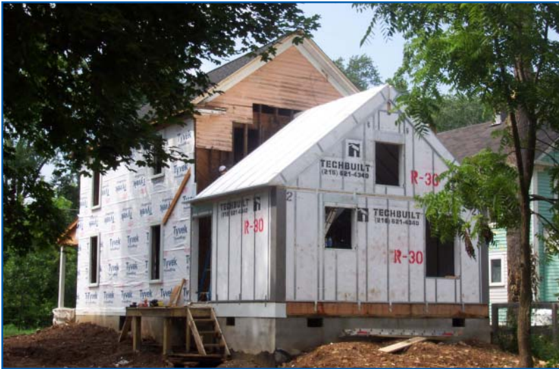
Addition constructed in 6 hours
