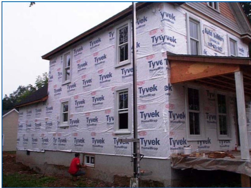
Air barrier on outside of house
