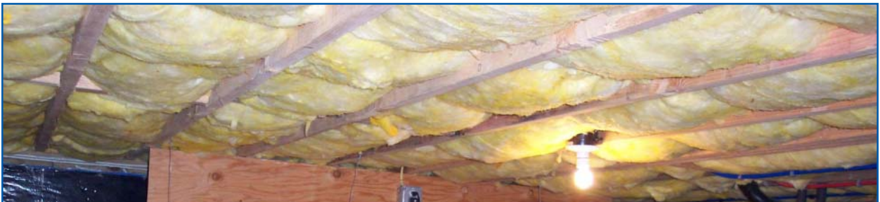
Floor insulation between joists
