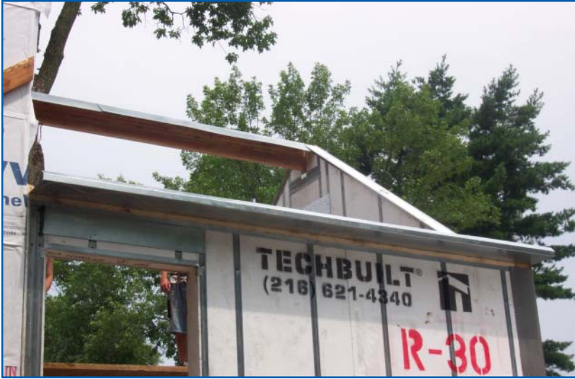
Ridge and eave supports for roof panels
