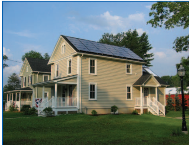
PV system on Cottage home
