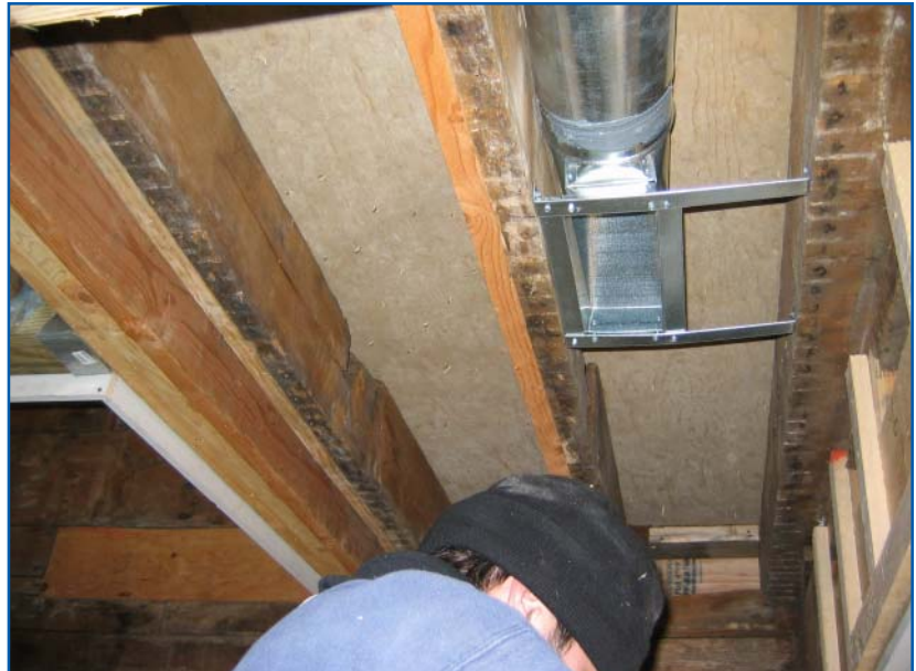
All duct joints sealed
