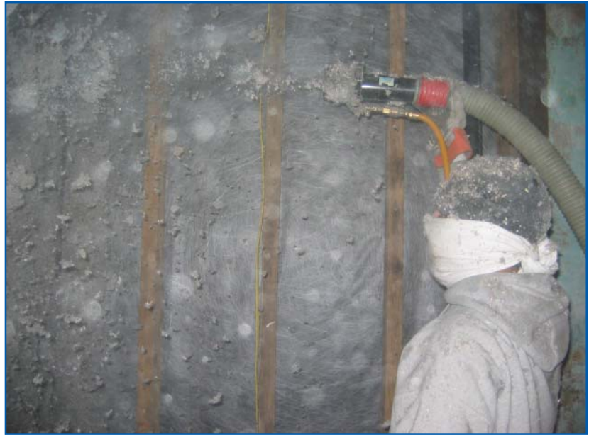
Blown cellulose insulation
