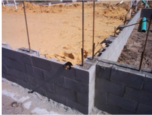
Insulated concrete forms the walls of the basement.
