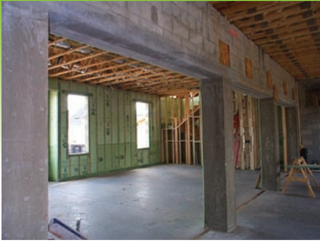
High foundation walls protect the home against groundwater and create an upscale profile.
