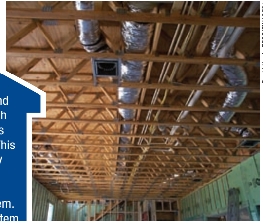
Open web joists were extremely useful for allowing the passage of ductwork within conditioned space.
