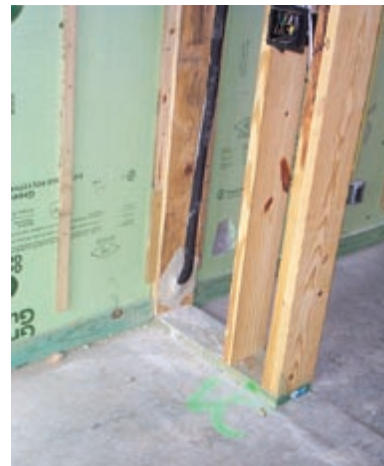
Sealing at all penetrations provides for airtightness in the building.
