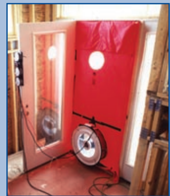
Home airtightness is tested with a blower door.
