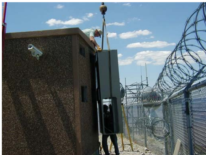
Jim Maclellan performs equipment maintenance at the Las Vegas 88D site.
