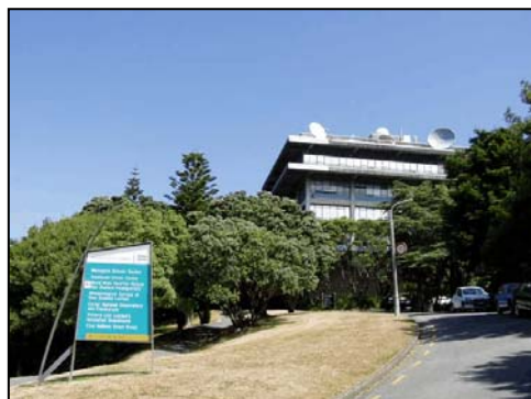
New Zealand's MetService Office in Wellington
