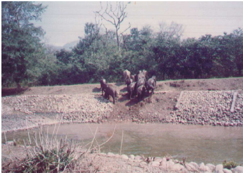
Fig.15-View of Water Tank for Elephants connected with the Chilla Power Channel
