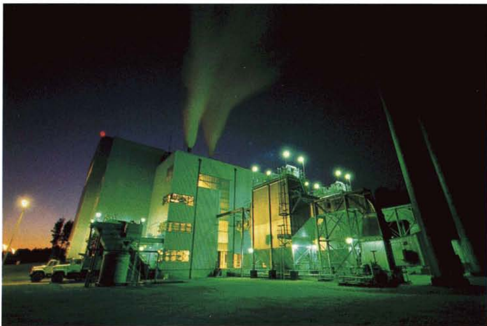
Shown above is the Refuse-fired Steam Generating Facility at Hampton, Virginia, a highly efficient trash-burning, energy-producing plant jointly developed by NASA, the Air Force and the City of Hampton. Effective air pollution control required development of an advanced electronic control system for the facility's precipitators, which remove pollutant particles from smoke.
