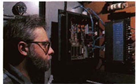
The spinoff electronic control system is in use at General Motors' Flint, Michigan plant (top). Above, a company technician is inspecting one of the installation's four control panels. The microprocessor-based control automatically senses changes in smoke composition and adjusts precipitator voltage and current to assure maximal removal of pollutant particles.
