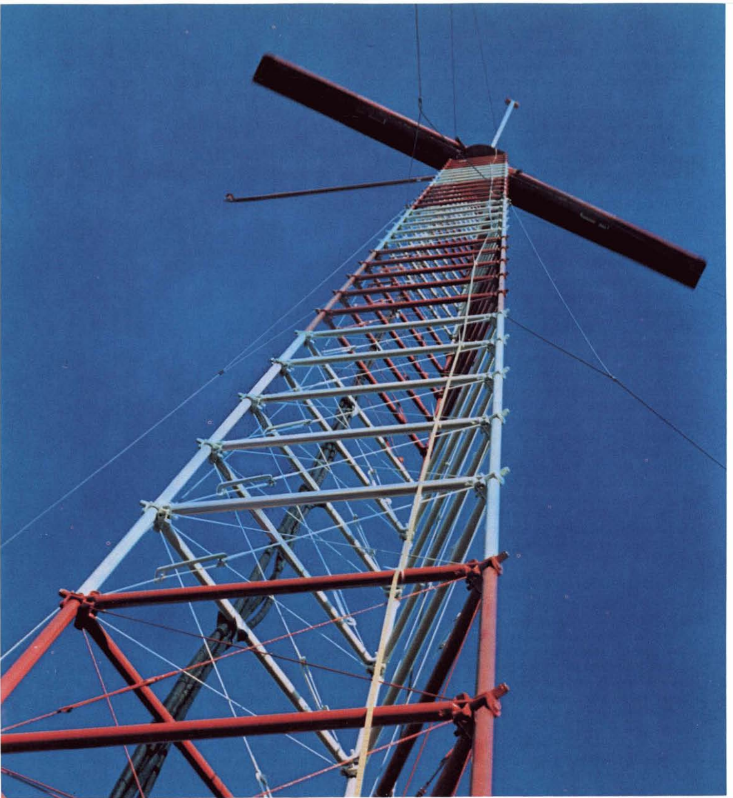
Reusable tower arrives on scene in collapsed form, then is extended 100 ft or more. A transfer from satellite antenna tower holds spotlights and speakers for outdoor concerts, among other uses.
