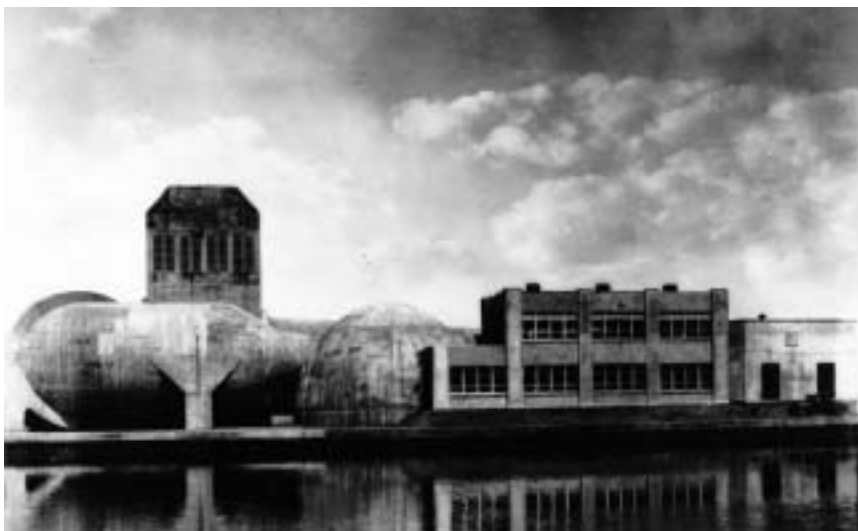
The 8-foot, high-speed wind tunnel at the NACA Langley Aeronautical Laboratory provided the means for testing large models and some full scale components at a simulated speed of 500 miles per hour.
