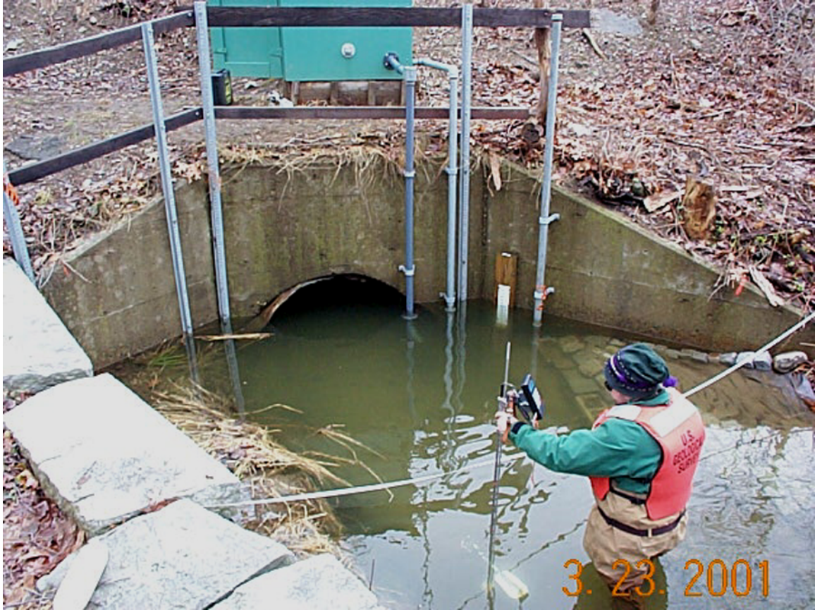
Measuring flow at Stony Brook culvert, Waltham, MA (photographer unknown).
