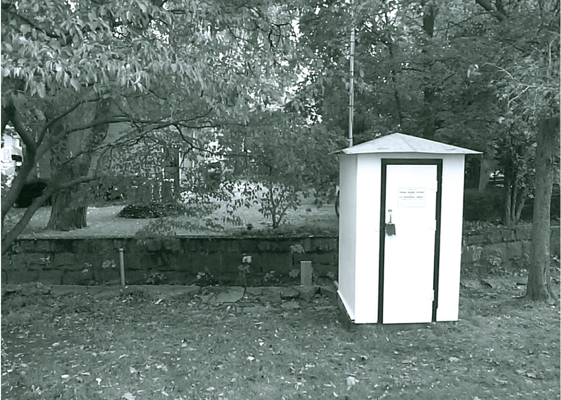
Town Brook at Quincy, Massachusetts, gaging station. (photo by J.L. Zanca)
