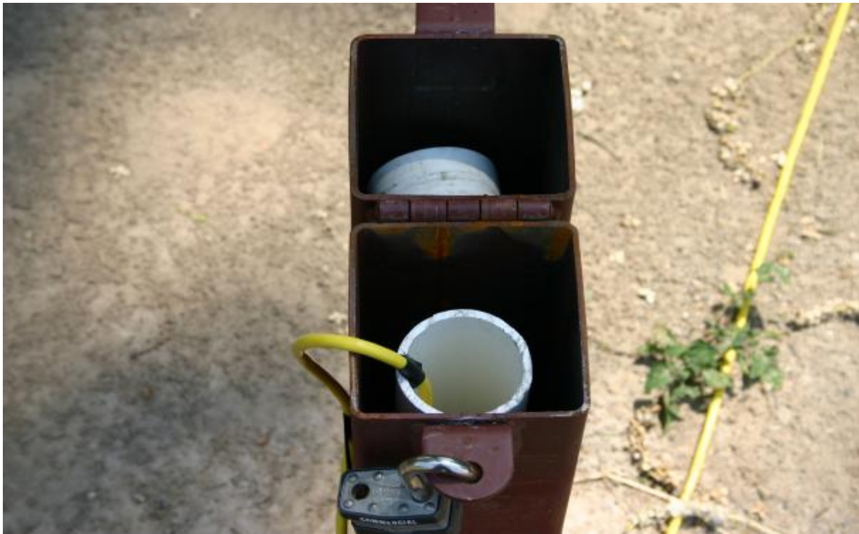
Top of observation well showing the top of the PVC well casing and the cable from the pressure transducer set in the well to measure the water levels.
