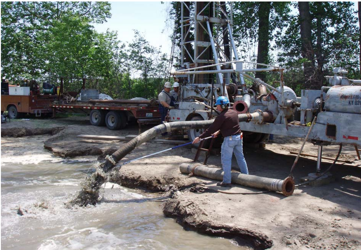
Hydrogeologist collecting drill cutting samples from test pumping well boring.
