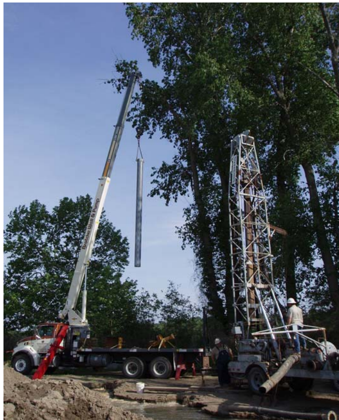
Well screen being installed in the test pumping well.
