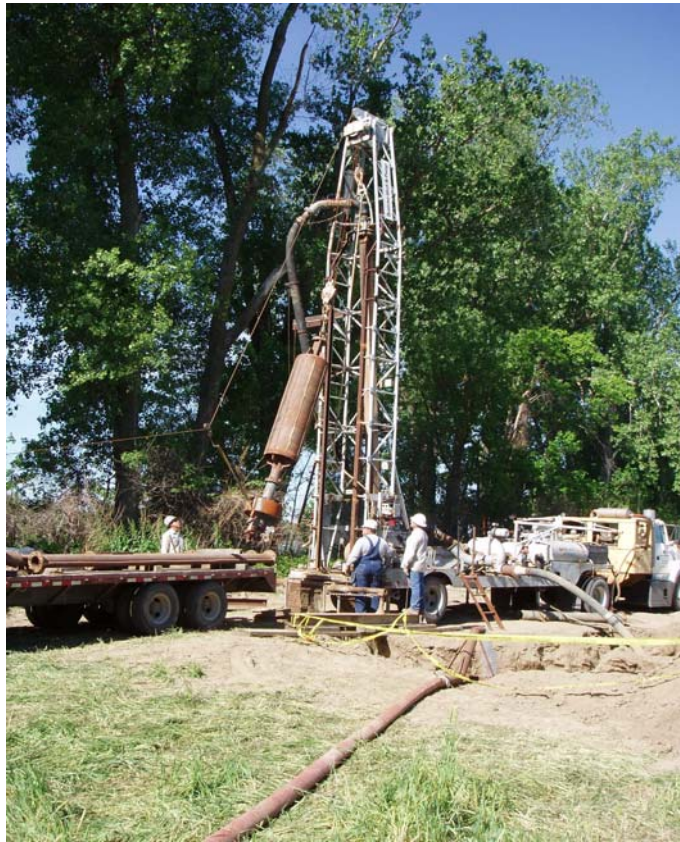
Lowering the drill bit assembly into the borehole.
