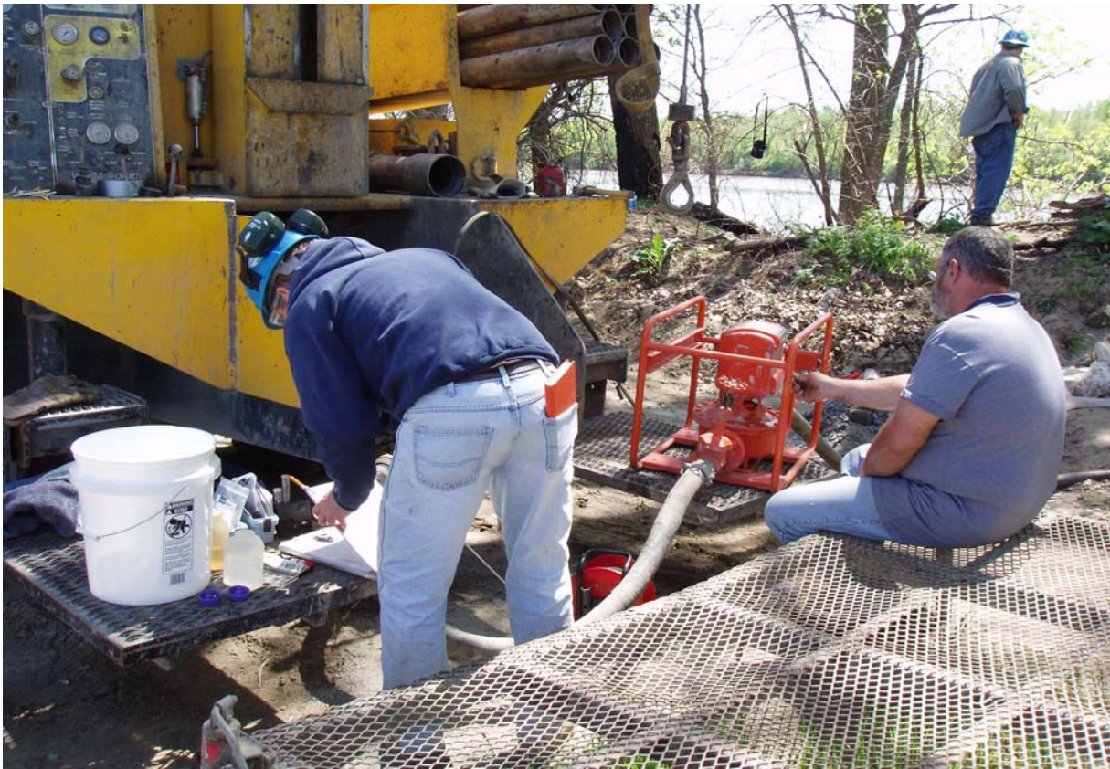
Conducting hydraulic interval pumping test at boring TB-06-2
