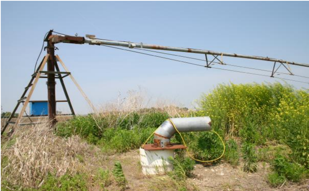
One of the irrigation wells in which water levels were monitoring during the aquifer test.
