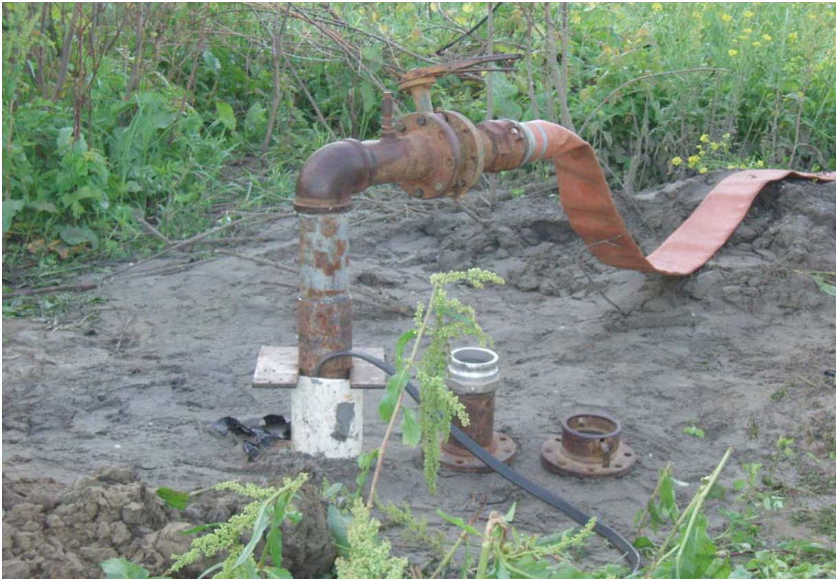
Temporary supply well for water to drill the test pumping well.
