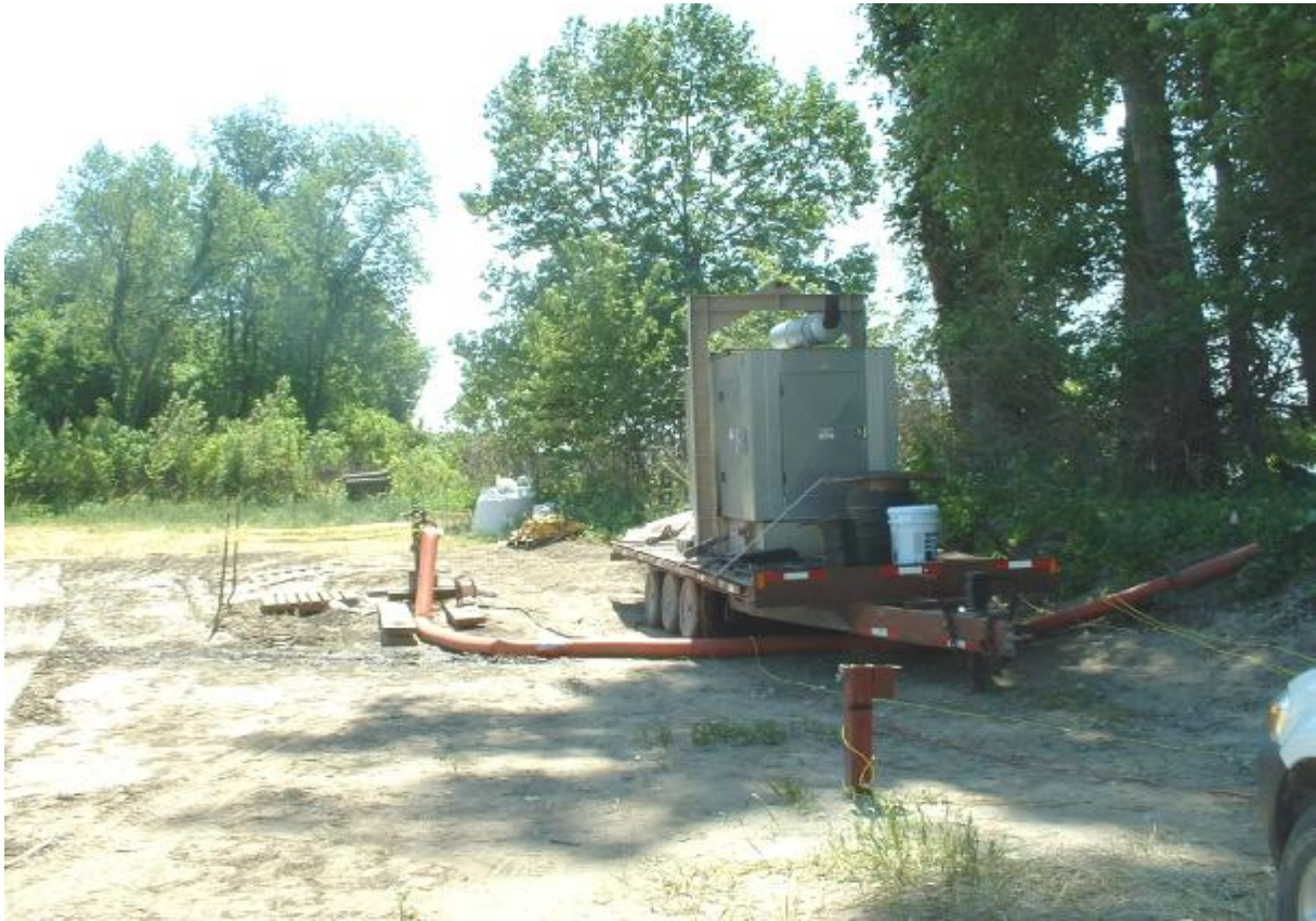
Test pumping well set up with temporary generator to power pump.
