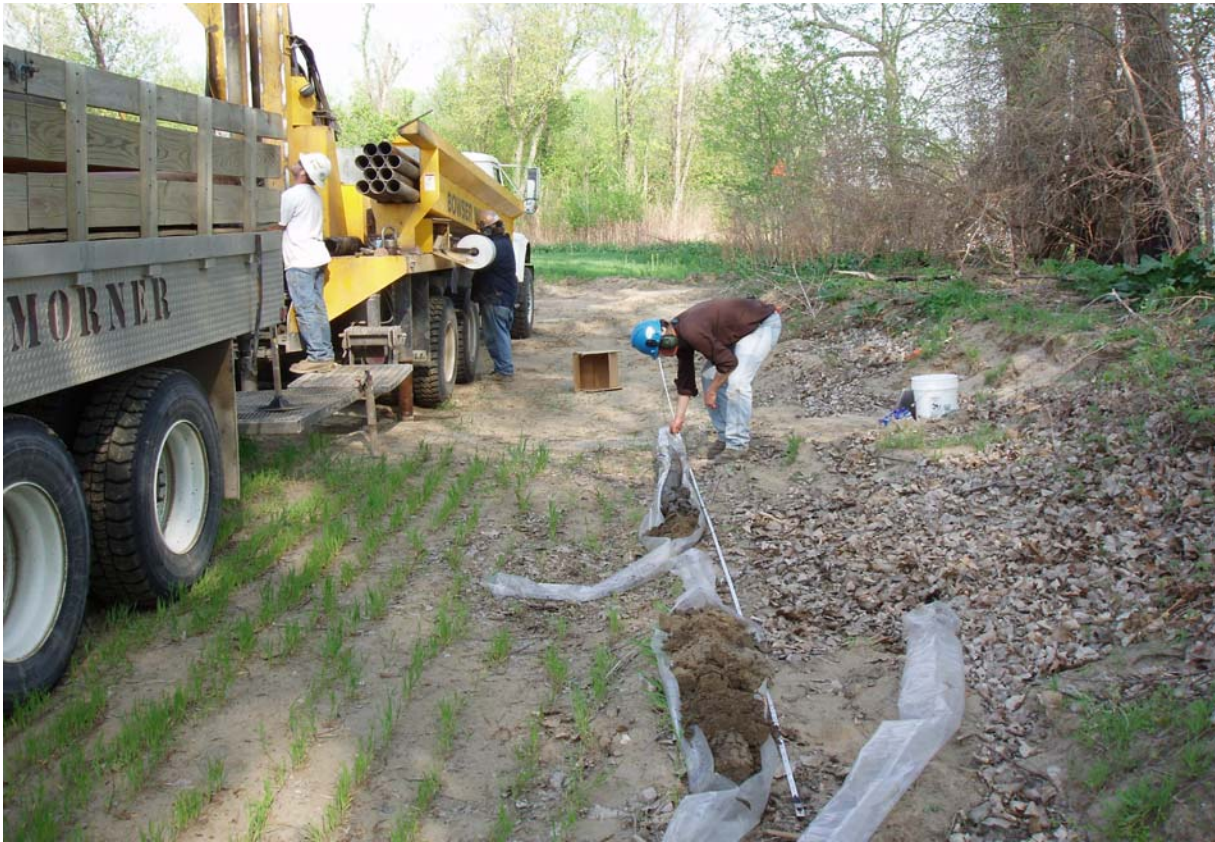
Hydrogeologist logging soil samples from the test boring.
