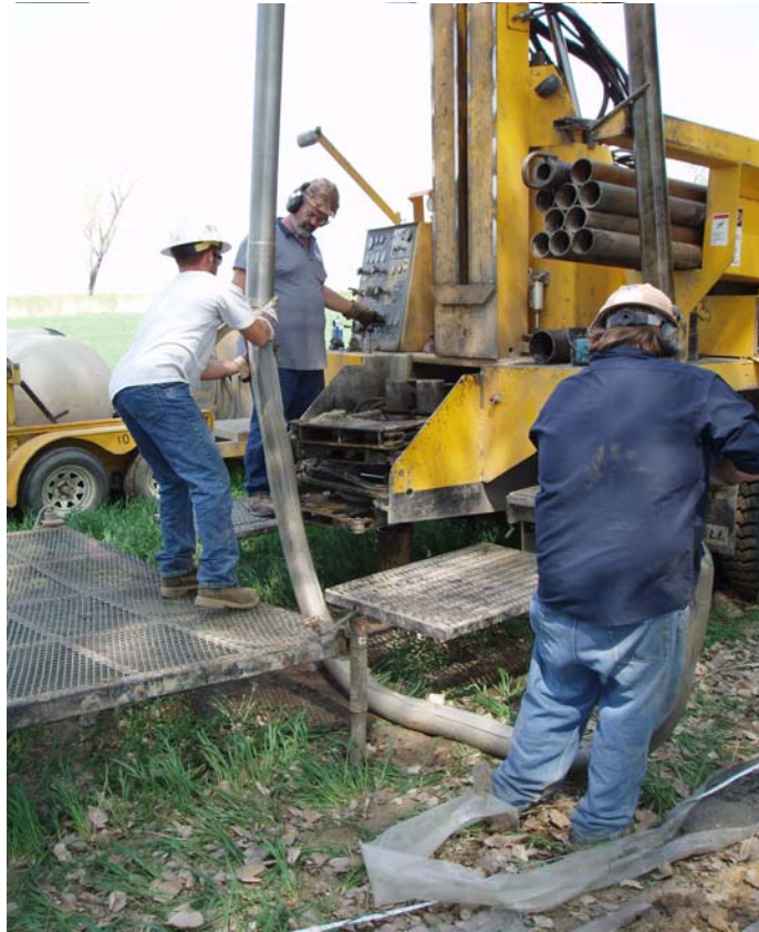
Drillers extracting soil samples from the rotasonic core barrel.
