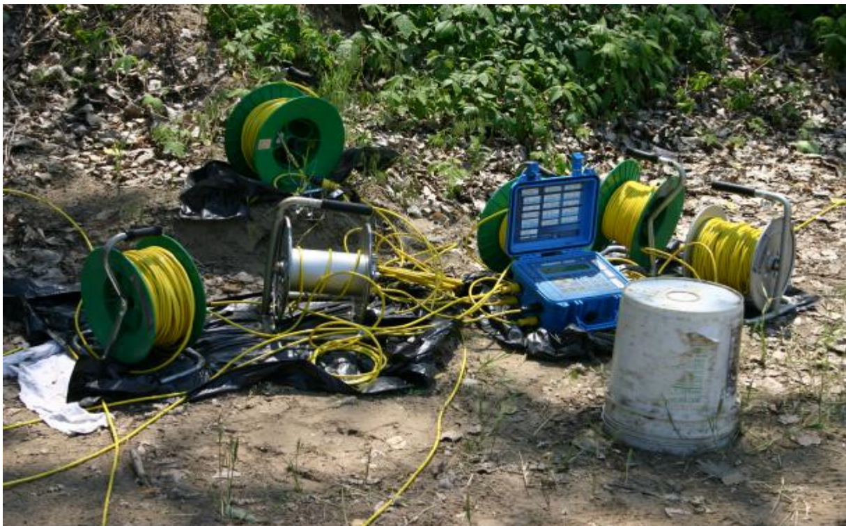
Water level data recorder that is connected to the cables from the pressure transducers installed in the pumping well and observation wells.
