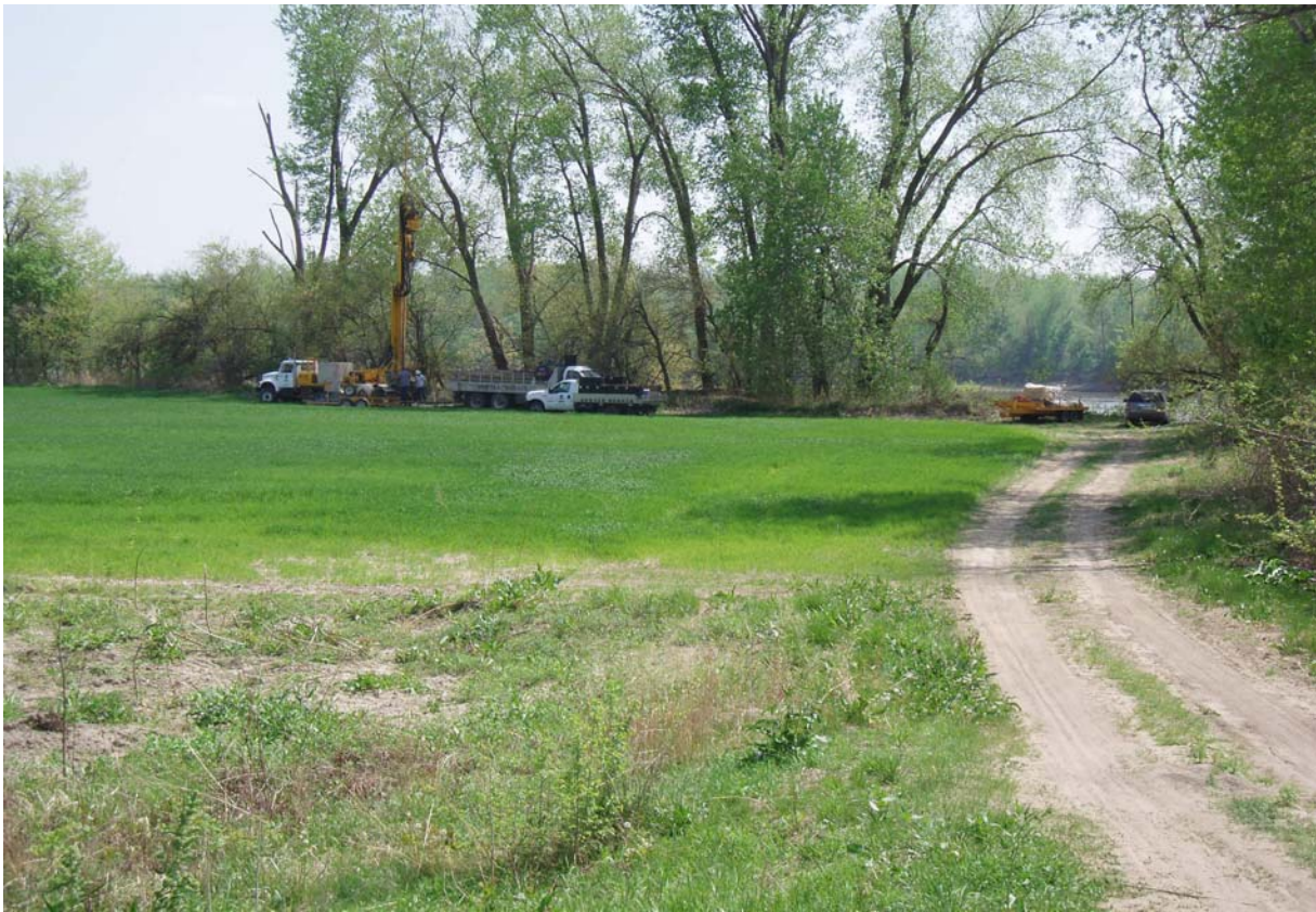
Rotasonic drilling rig set up at the first test boring TB-06-1
