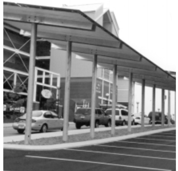
Eleven canopies over the parking lot at Finley Stadium in Chattanooga serve a dual purpose—they provide covering for fans attending sports events there, and they also generate solar-powered electricity for the Tennessee Valley (see story inside).
