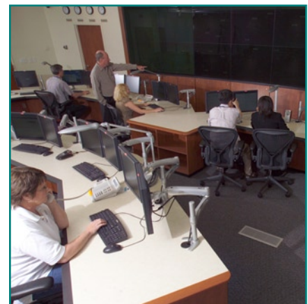
The EIOC provides a testbed environment for the latest operational techniques and grid technologies.
