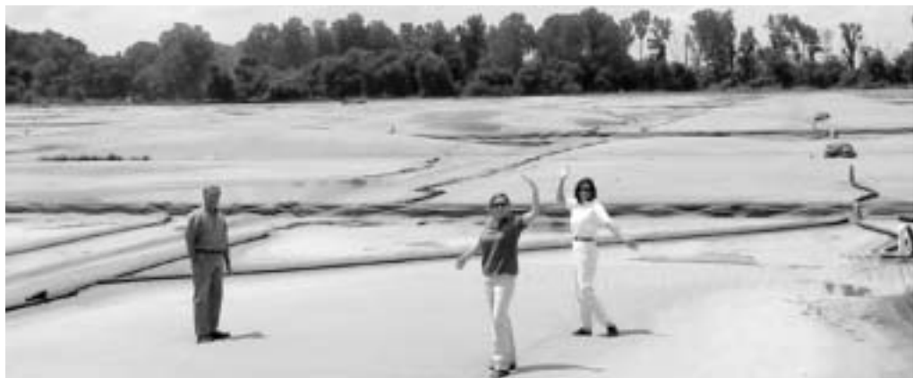
From left: Peter Alfonso, manager of the Memphis wastewater treatment plant, and Carmen Ledbetter and Angela Hamlin of Green Power Switch examine the plant's covered lagoon, where methane is captured.
