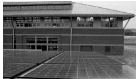
The MSU Landscape Architecture Building becomes the fifteenth GPS solar site.
