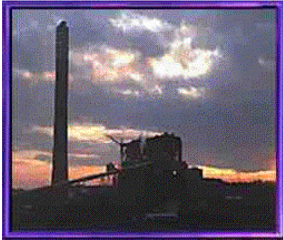
NTPC's 1000-MW Rihand Power Plant
