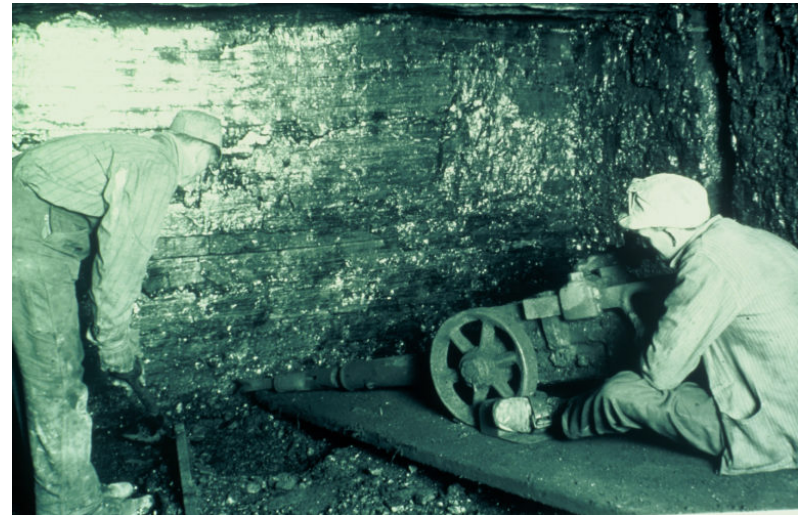
Drill and Blast
