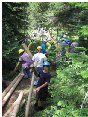
Above: Students are constructing a buck-and-rail riparian enclosure fence.
