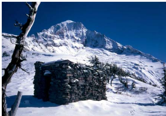
Mt. Hood Wilderness Timberline Winter Trail Shelter
