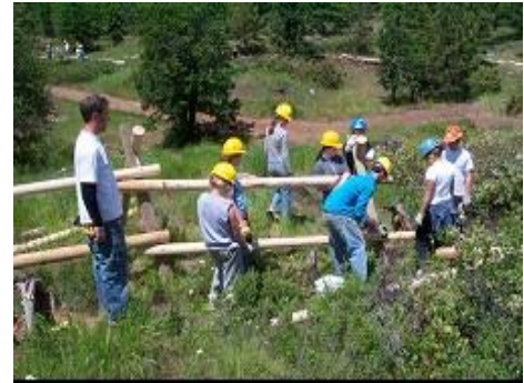
Photo above: Catlin Gabel School students participate in building a buck-and-rail fence to exclude cattle from grazing along Wildcat Creek.
