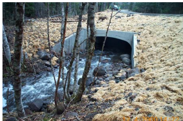
After (with erosion control)
