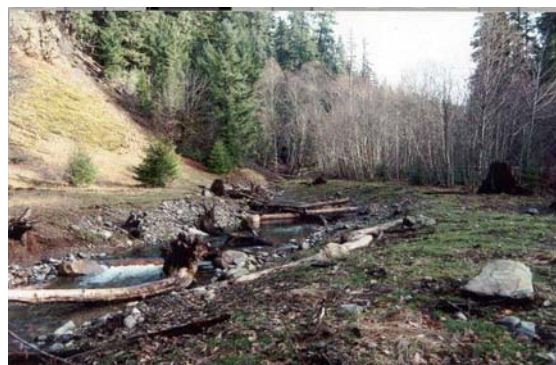
After - reconnected to river and side channel excavated
