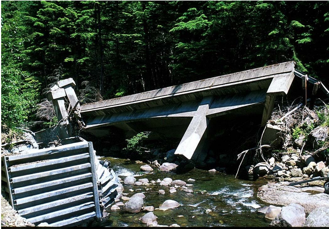
Wash Creek Bridge, Fish Creek Watershed, Clackamas River, Oregon.
