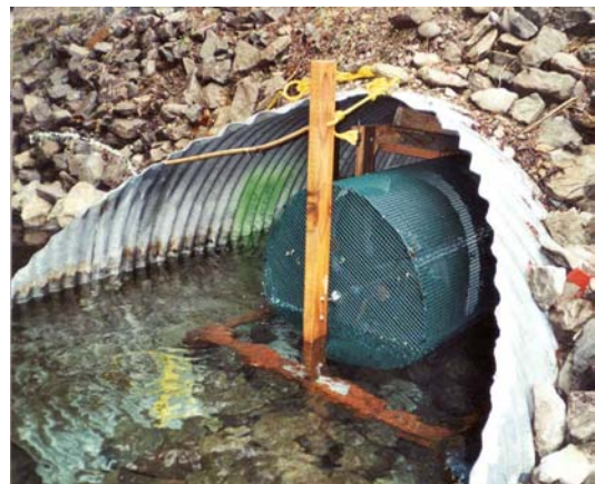
This two-way culvert trap is used to monitor movement of juvenile fish in and out of a side channel. The project is sponsored by OBOB's with watershed council support
