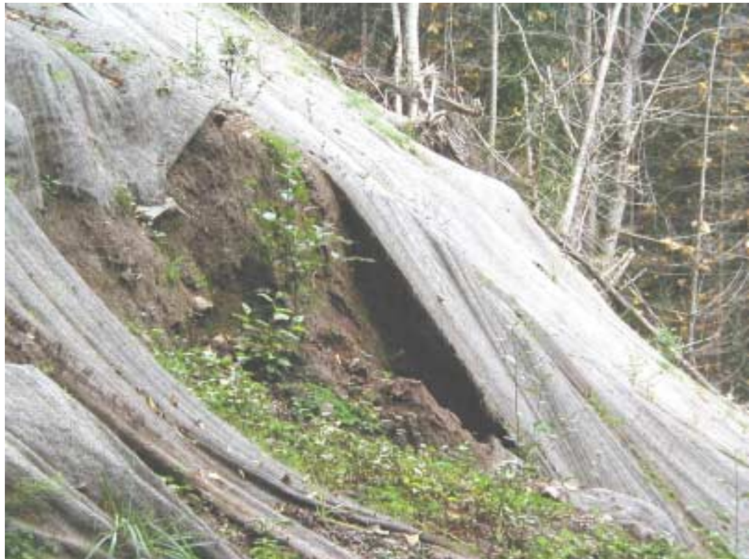
Figure 19. Poor vegetation establishment resulting from steep stream banks, use of plastic woven material and lack of moisture during the dry season.
