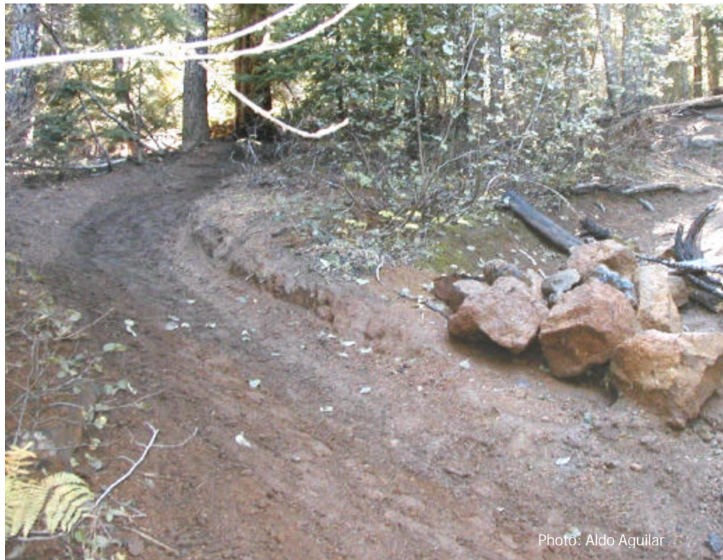
Figure 23 - Trail reconstruction relocated a popular trail around steep, eroding soils
