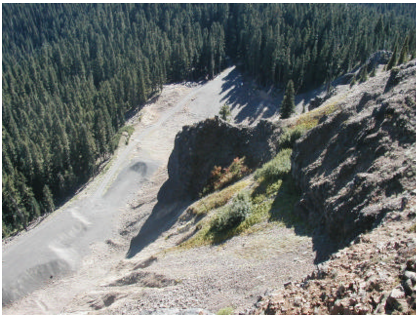
Figure 14 - Quarry and gravel stockpile area at base of Steamboat Mountain, 2002
