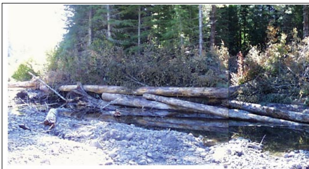
Figure 32. - Photo of large wood revetment at Trout Creek (river mile ~ 7.3).
