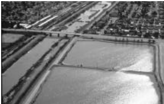
Figure 21: Artificial recharge in Santa Ana riverbed. Artificial groundwater recharge in the Santa Ana Riverbed, Orange County Water District, California. Source: Orange County Water District.
