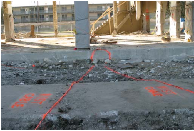
Figure 23. Cables on east side of building. Cables were run from the transmitter site under the building to the east side of the building.
