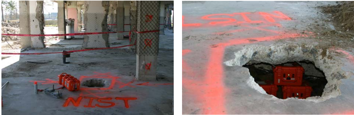
Figure 18. Fixed transmitter location in hole in concrete on bottom floor.
