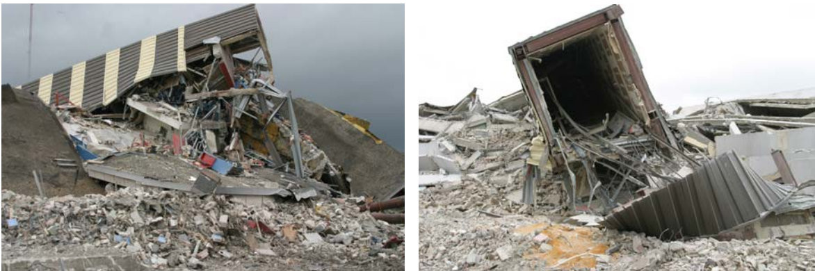
Figure 71. Location of the elevator shaft and transmitters after the implosion.
