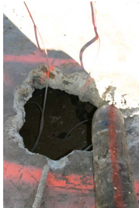
Figure 23. Cables on east side of building. Cables were run from the transmitter site under the building to the east side of the building.
