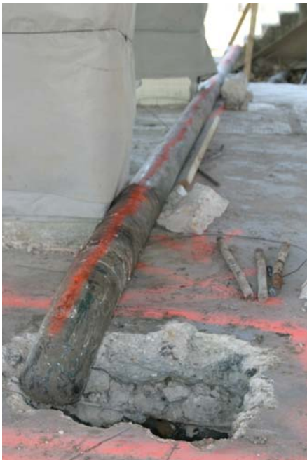
Figure 23. Cables on east side of building. Cables were run from the transmitter site under the building to the east side of the building.
