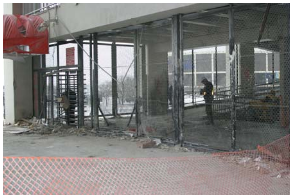
Figure 3. Pre-implosion preparation inside the stadium.
