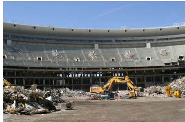
Figure 2. Pre-implosion deconstruction of the stadium.
