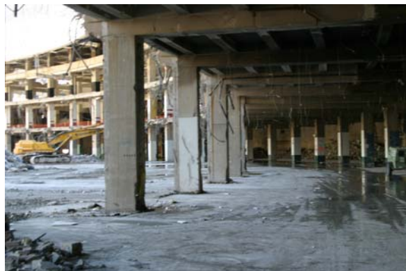
Figure 3. Pre-implosion preparation inside the stadium.
