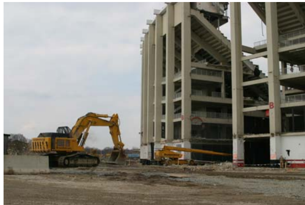
Figure 2. Pre-implosion deconstruction of the stadium.
