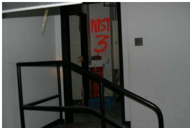
Figure 18. Fixed transmitter location TX 3; an intermediate level (office area) of the convention center.
