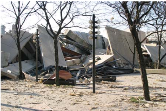
Figure 81. Photos of partially collapsed convention center after the implosion.
