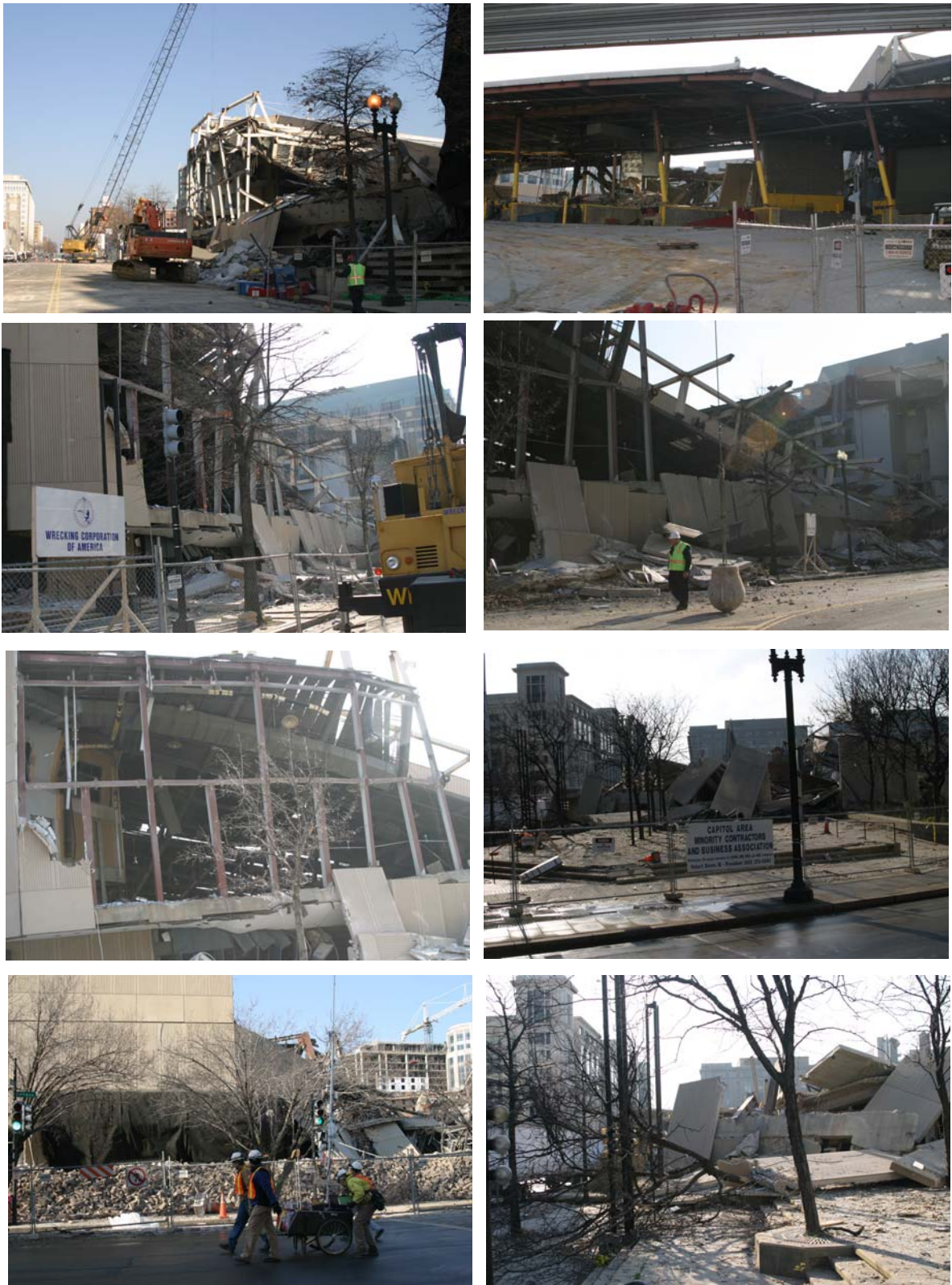
Figure 82. Photos of partially collapsed convention center after the implosion.
