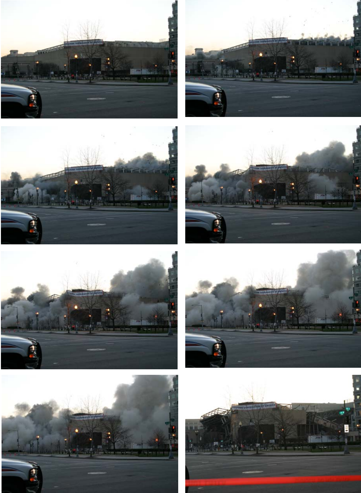
Figure 80. The convention center collapses during the implosion sequence.
