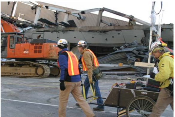
Figure 81. Photos of partially collapsed convention center after the implosion.
