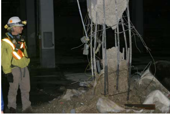
Figure 3. Pre-implosion preparation inside the convention center.
