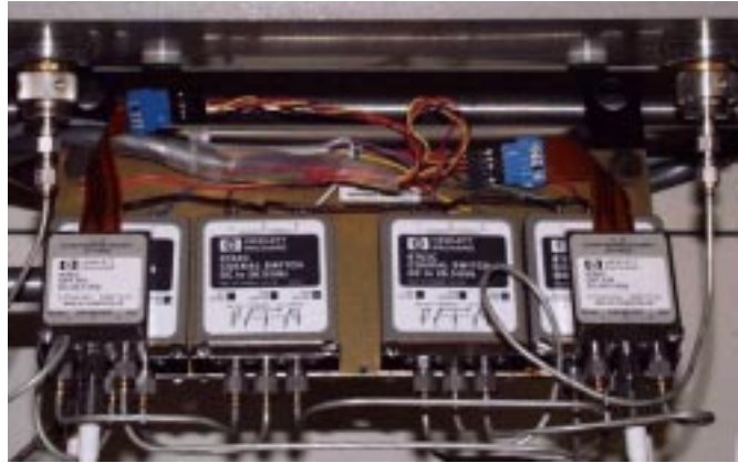
Figure 3. Coaxial switch matrix that implements the four-port system shown in Figure 1. Measurement range is 50 MHz to 26.5 GHz.
