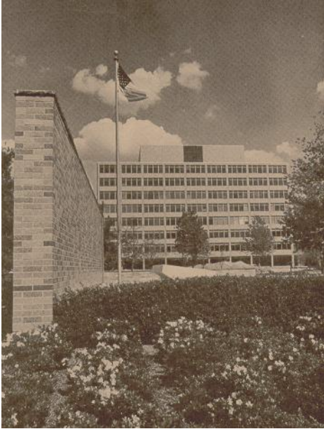
SSA's East High Rise Building on Security Blvd. was built in 1970. HCFA personnel moved into the EHR and other nearby buildings.
