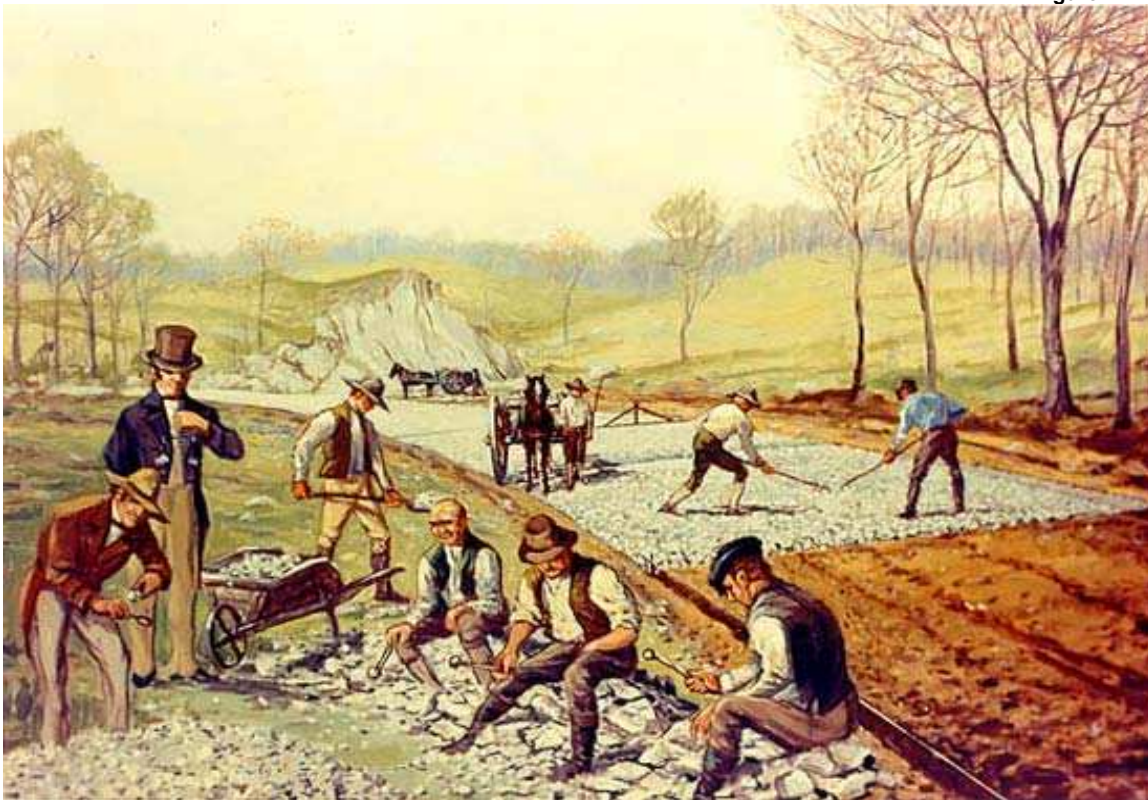
Penetration Macadam is an early form of modern-day blacktop in which the paving is built-up by layering crushed stone with applications of tar.
