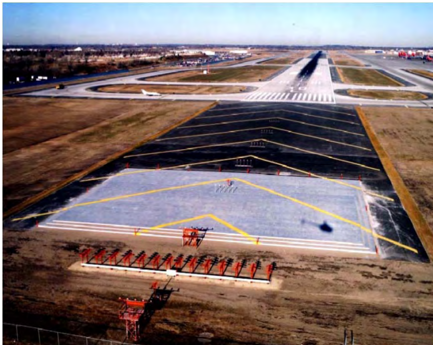
FIG AD 1.1-51 Engineered Materials Arresting System (EMAS)
