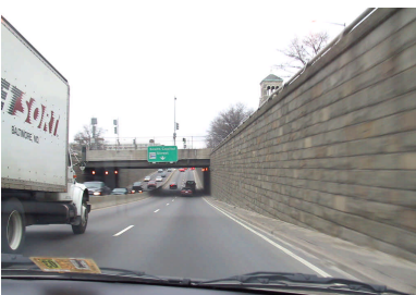
M street underpass
