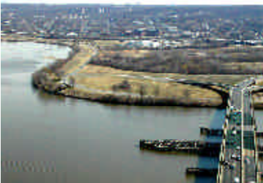
Parkland at Poplar Point
