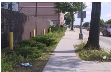
Sidewalk conditions near O Street SW
