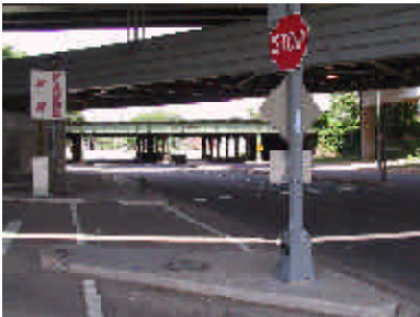
South Capitol Street below I-395
