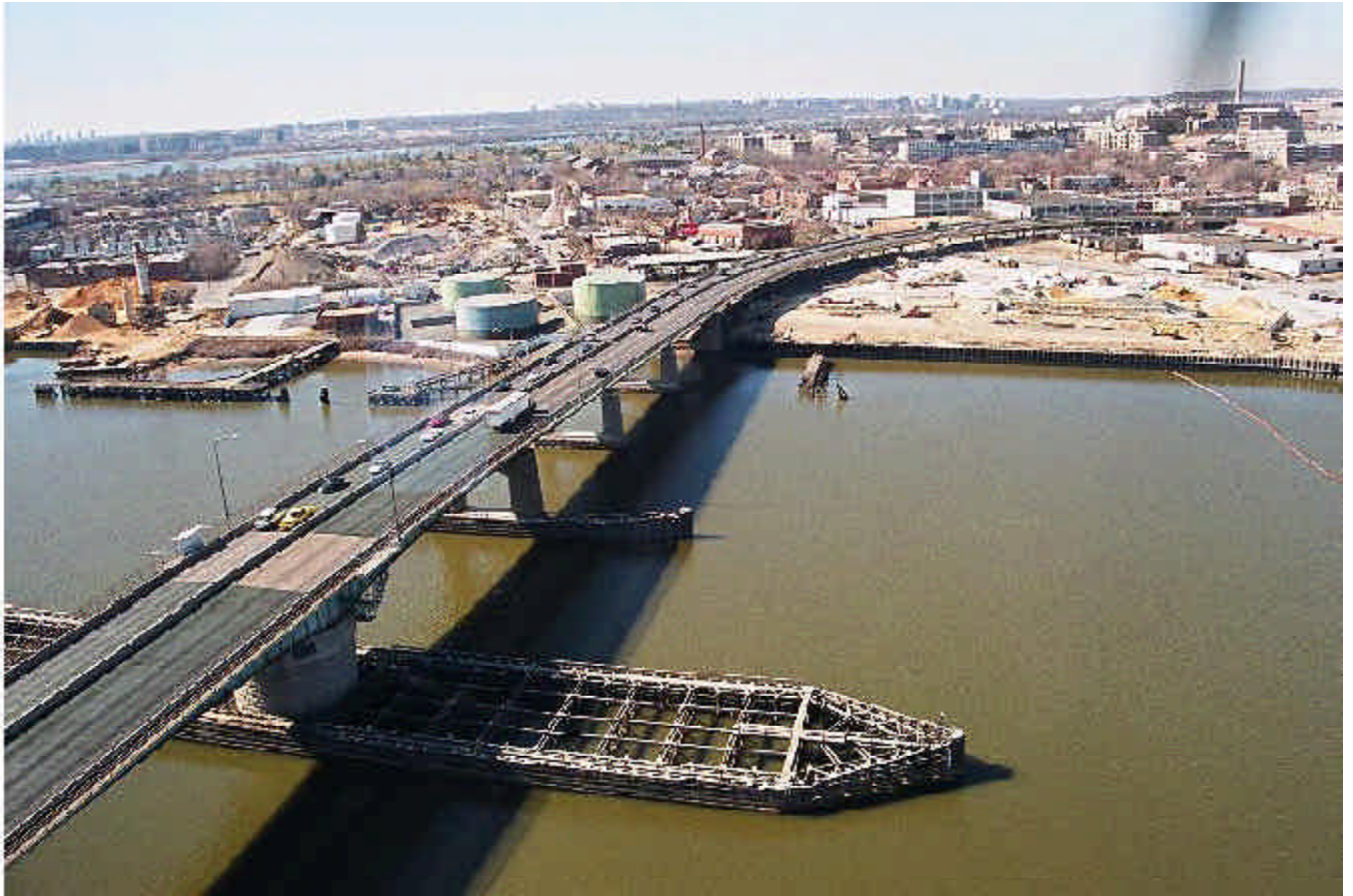
The height of the Frederick Douglass Bridge increases the length of ramps connecting to city street grid
