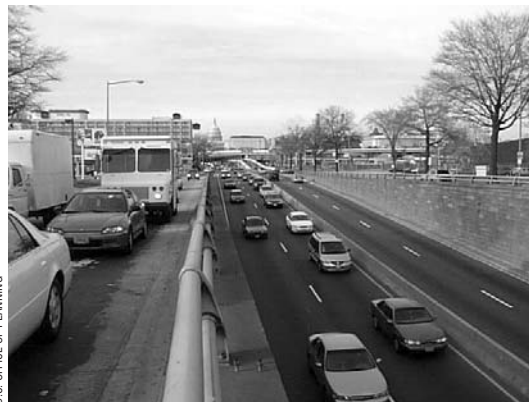
South Capitol Street, used as a commuter thruway, passes under the M Street intersection; service lanes carry local traffic at grade.
