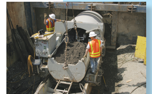
Spoils removal from a microtunneling operation.
