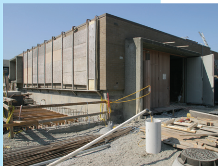
A pump station under construction.
